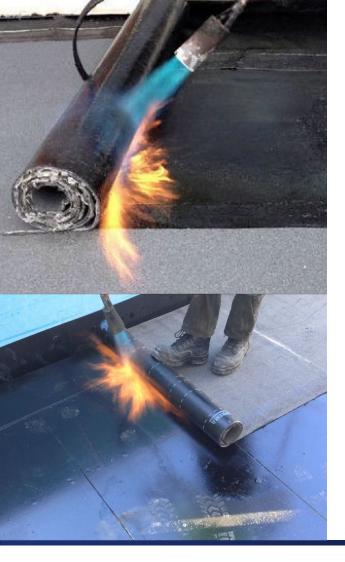
• Modified bitumen sheet applied by open flame to of the left ... with a release sheet covering it. The backside of sheet and subsequently adhere to convert structure, as the release sheet is removed (see photo) ... and adhered to the
